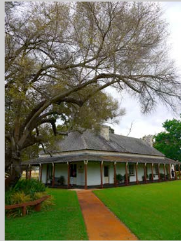
View of homestead, Wonnerup Precinct. Image © Office of Heritage, Western Australia 2011.
